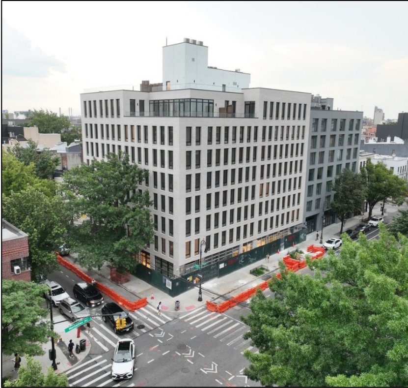
170 Freeman Street, Greenpoint (68 units)
