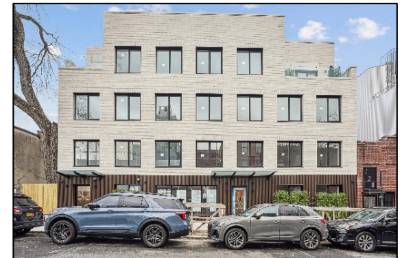
132-134 Waverly Avenue Clinton Hill (15 units)
