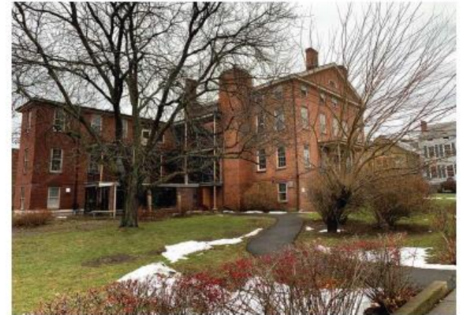
Existing Conditions - Exterior
