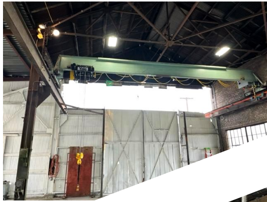
Left: Gantry crane repair - spanning entire workshop to loading dock.
