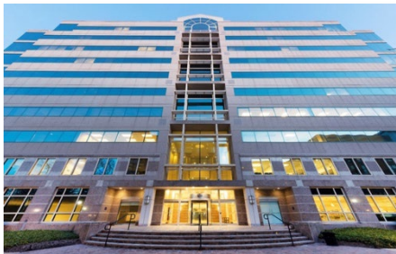
Argon Plaza Office in Fairfax, VA currently zoning to convert parking lot to apartments
