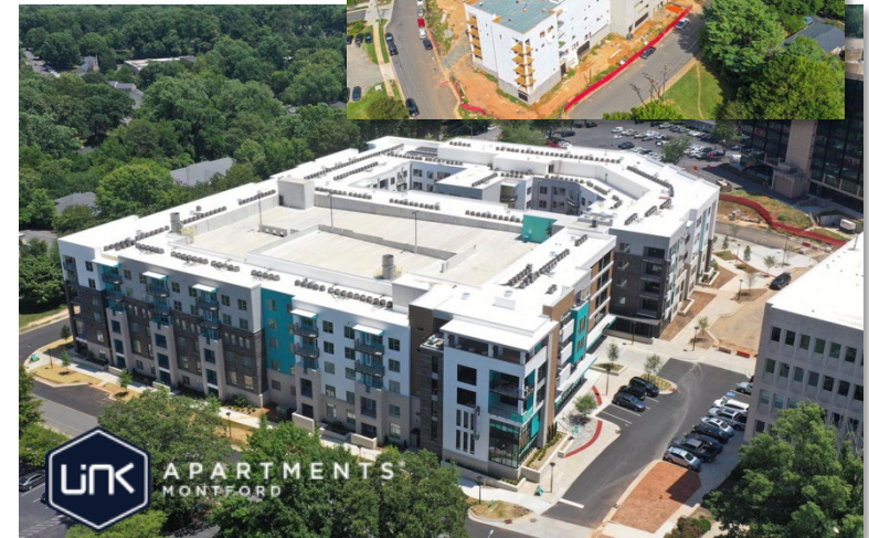
Link Apartments SM Montford constructed on the surface parking lots of 4601 Park Rd and 1515 Montford Park office buildings
