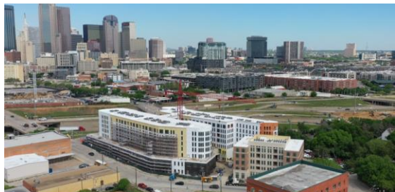
The Ambassador, Dallas (Under Construction)
