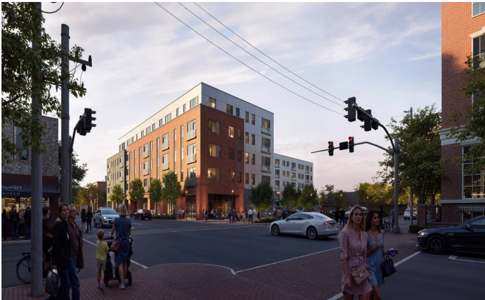
Cameron Square, Winchester (Under Construction)
