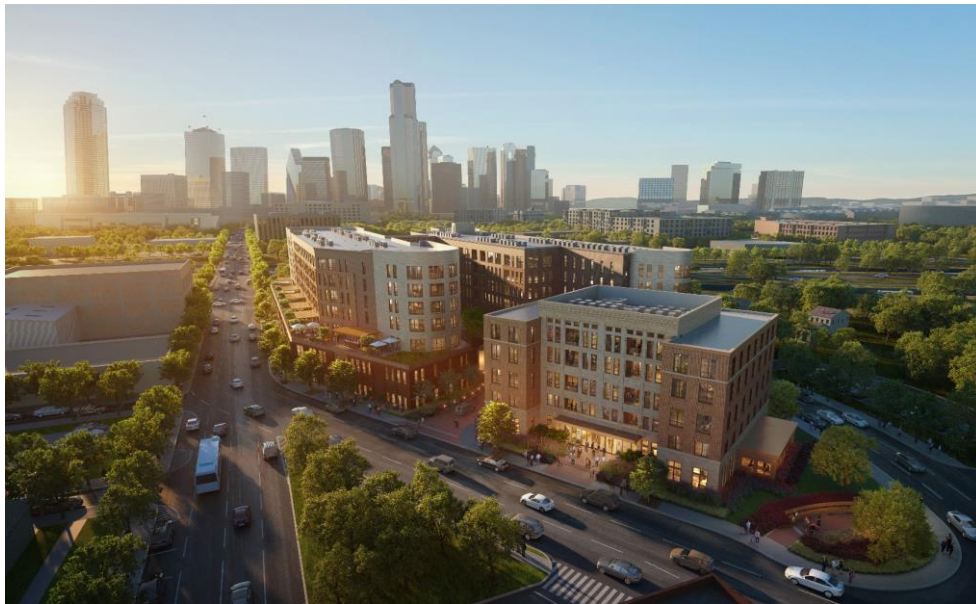
The Ambassador, Dallas (Under Construction)
