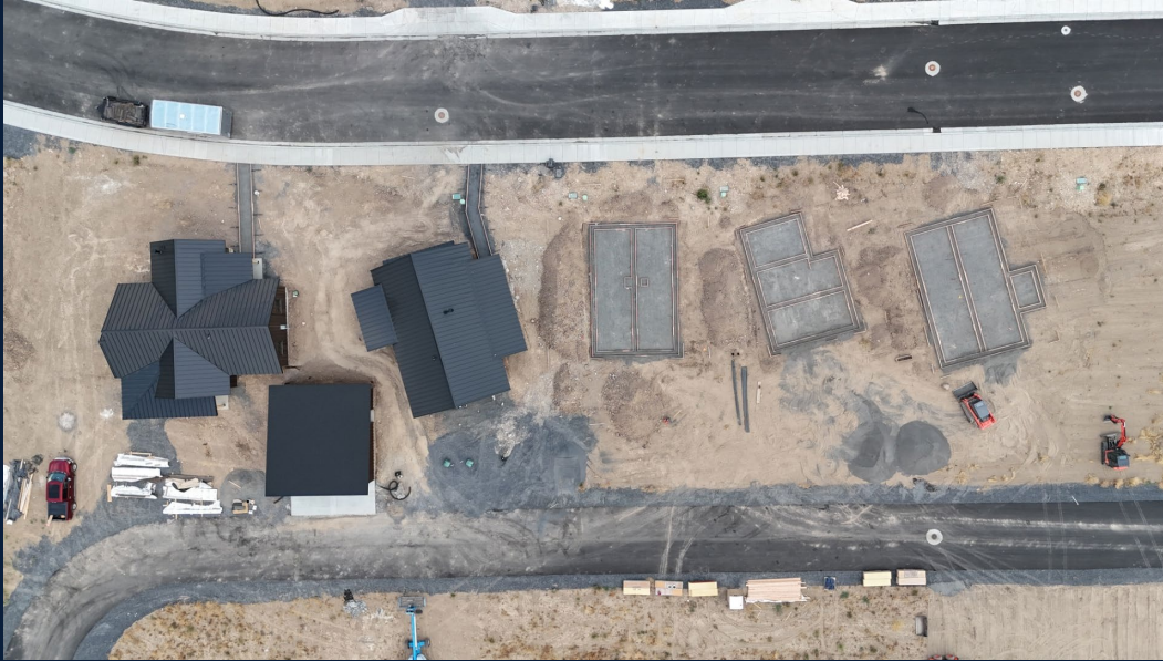
July 22, 2026 — Lot 17 complete (left). Lot 16 foundations poured (right).
